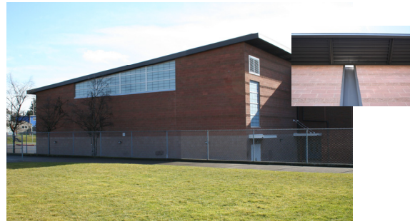
NORTH EVERETT MIDDLE SCHOOL GYM • Everett, WA Phillip Lehn Project Architect, NAC | Architecture • Seattle
