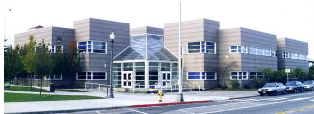
EVERETT HIGH SCHOOL SCIENCE BUILDING • Everett, WA Phillip Lehn, Project Architect, Botesch, Nash & Hall
